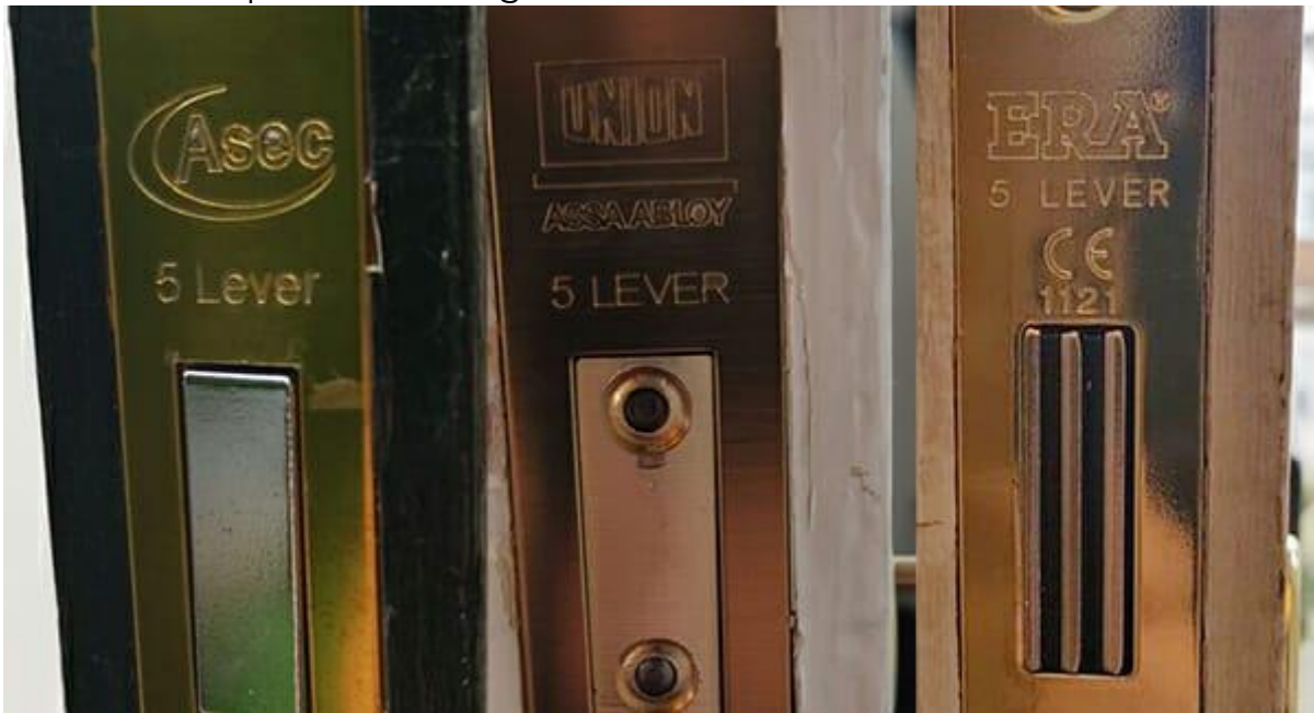
Number of 5 Levers stamped on Faceplate of Lock
