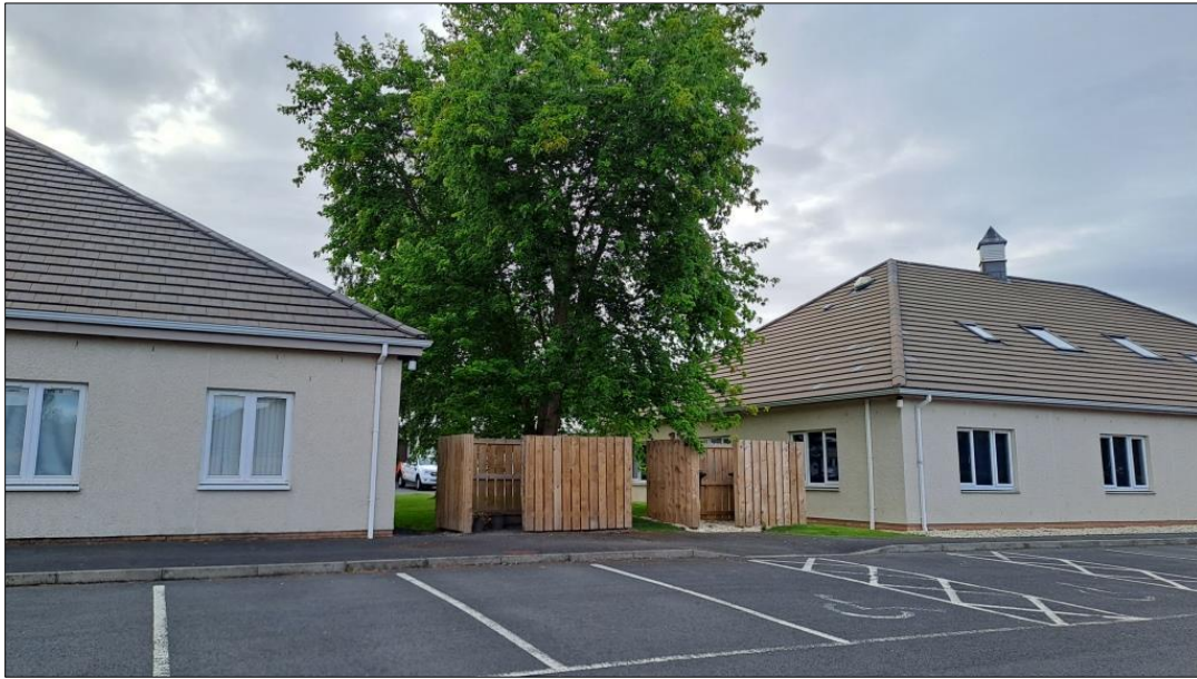
Fig 7: Bin store adjacent to north elevation.
