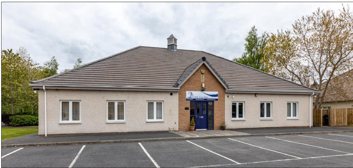
Fig 1: East elevation of 3 Rowan Court
