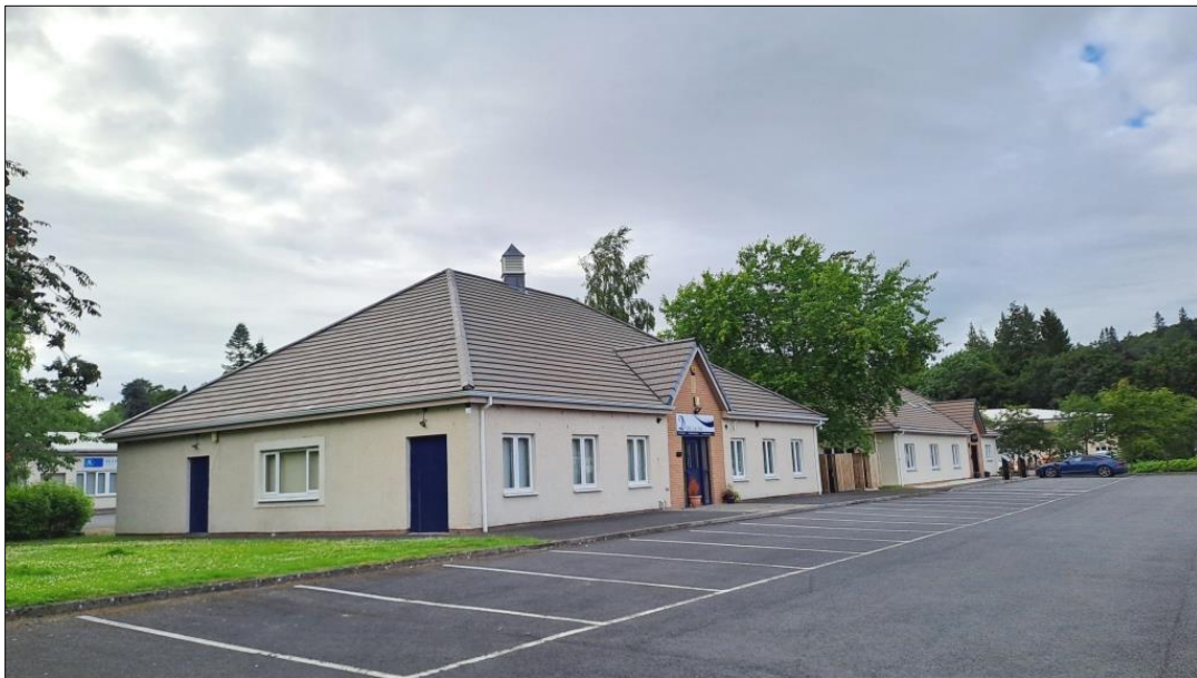
Fig 6: South and east elevations and parking
