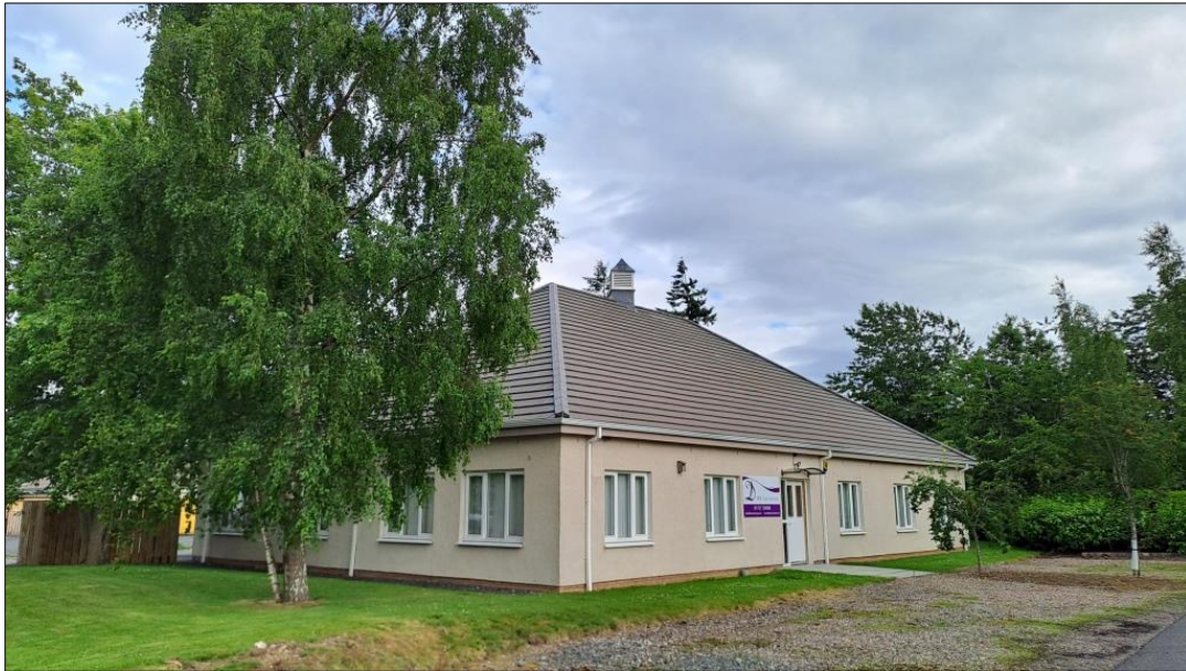
Fig 3: North and west elevations
